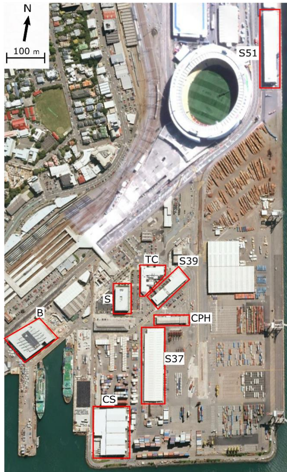
Figure 5.47: CentrePort Wellington map identifying buildings studied in this reconnaissance. (Base image from Google Earth™)
