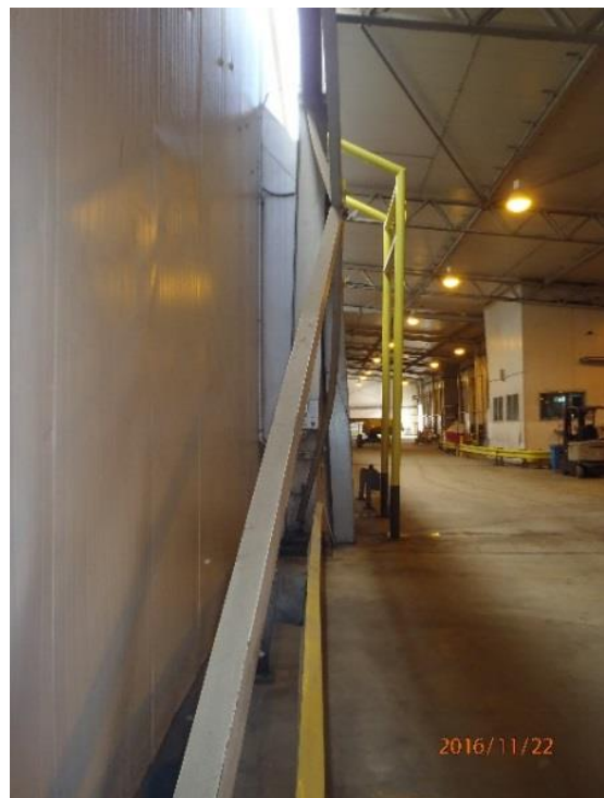
Figure 5.67: Internal east wall in northern part of the Shed, which shows column-pedestal connection failure due to rotation of the base of the column and buckling of concentric bracing. (Approx. at S41.280939° E174.784778°, taken at 1615 hrs on 22NOV16)
