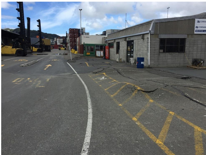
Figure 5.77: Looking south along western-most row of piles from partially demolished and buried Pipitea Wharf, which is approximately 16 m west of Building S37. Fill settled 300 mm relative to embedded piles (S41.278798°, E174.785186°, taken on 17NOV16). A cross section (LT1) is shown in Figure 5.29.
