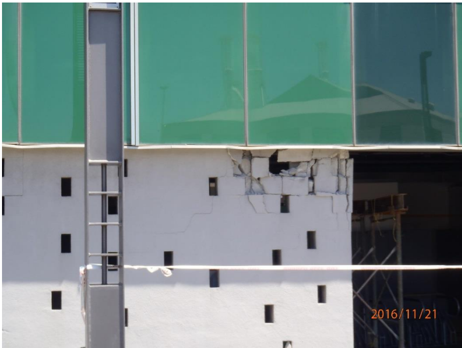
Figure 5.81: Damage to ground floor infill wall on the east side of the S building (S41.278114°, E174.784715°, 1241 hrs on 21NOV16)
