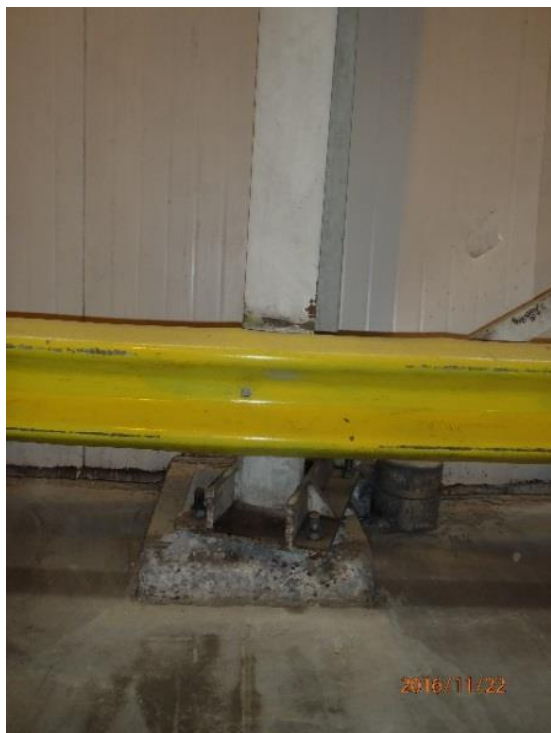
Figure 5.67: Internal east wall in northern part of the Shed, which shows column-pedestal connection failure due to rotation of the base of the column and buckling of concentric bracing. (Approx. at S41.280939° E174.784778°, taken at 1615 hrs on 22NOV16)
